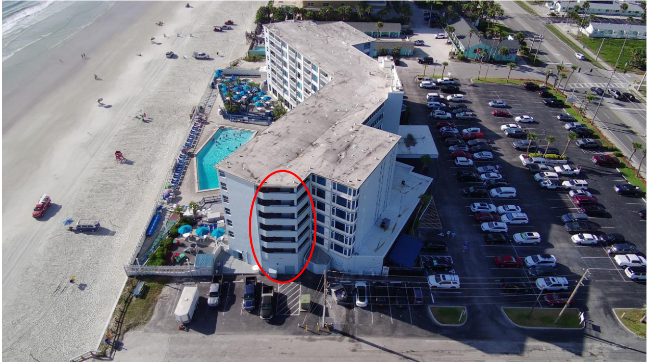
Photograph #3 – North building elevation (North walkway corridor with significant damage circled)
