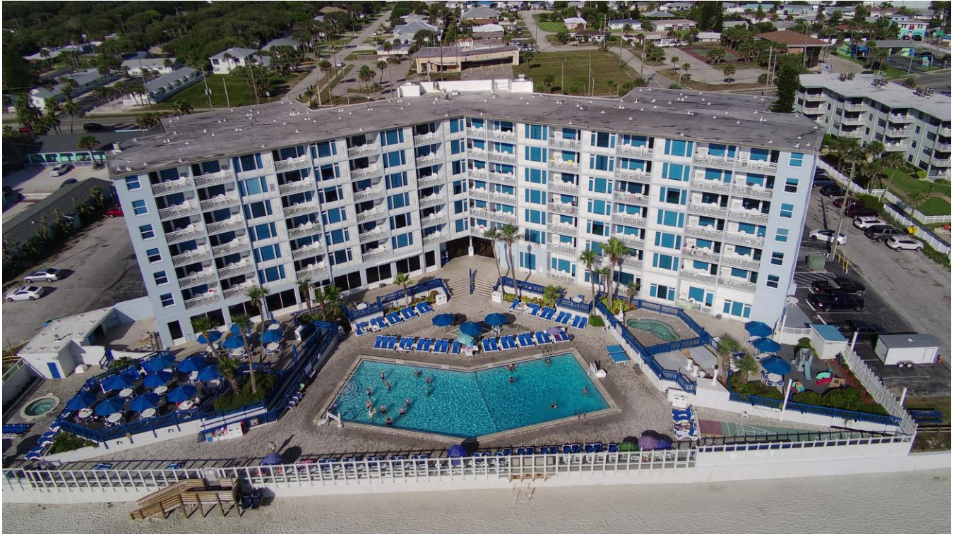
Photograph #1 – East building elevation
