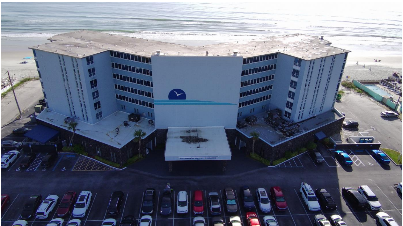
Photograph #2 – West building elevation
