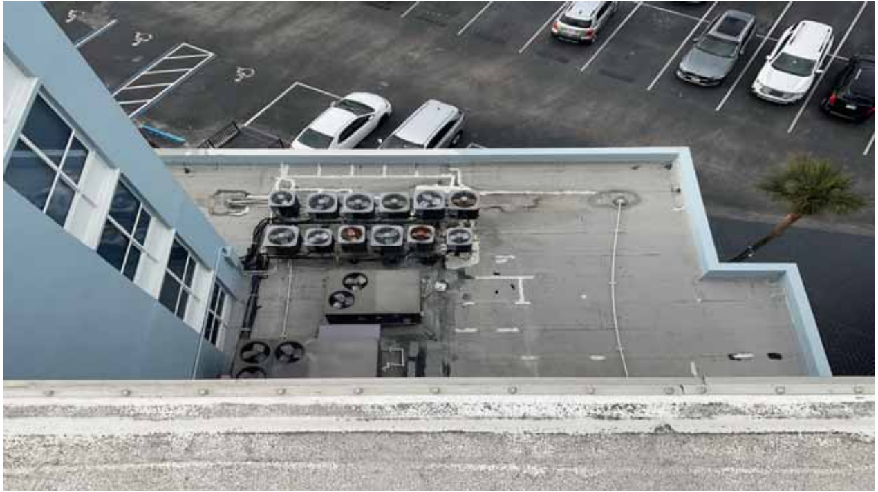
Roof - Lower South
