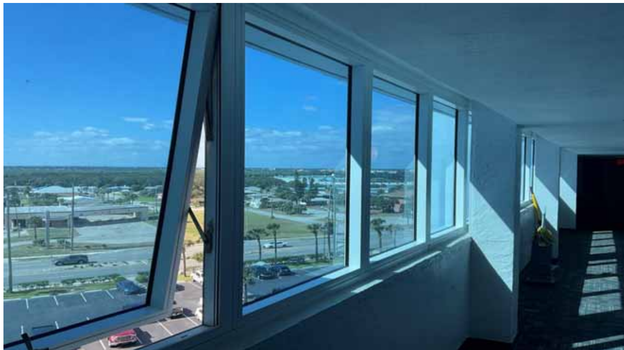
Hallway Windows - Typical
