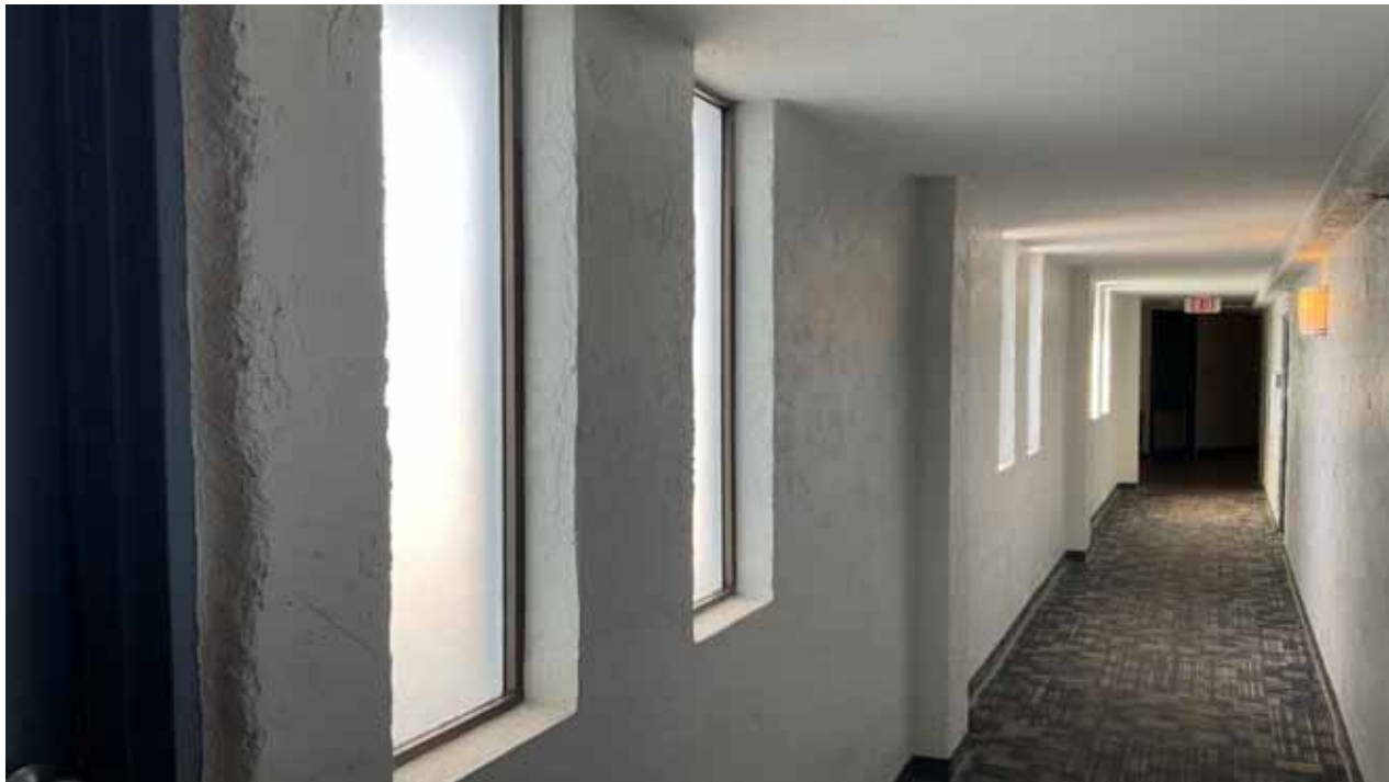
Hallway Windows - Level 2
