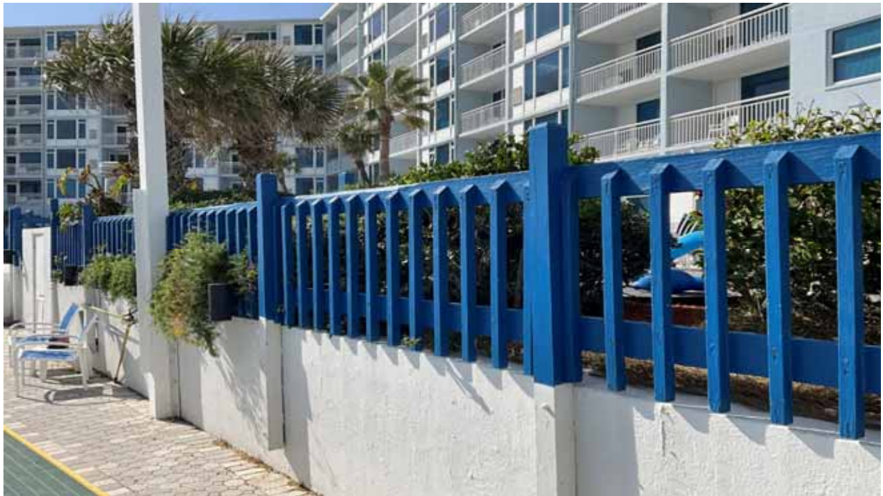
Fence/Railing - Pool Deck
