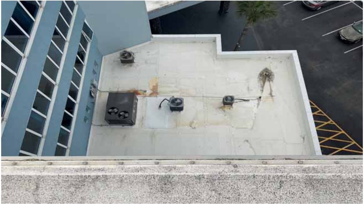
Roof - Lower North
