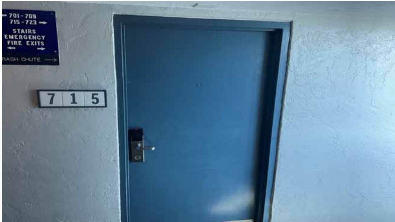
Unit Entry Door - Typical
