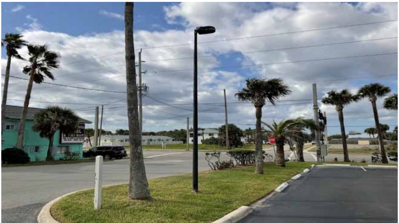
Lighting - Parking Lot
