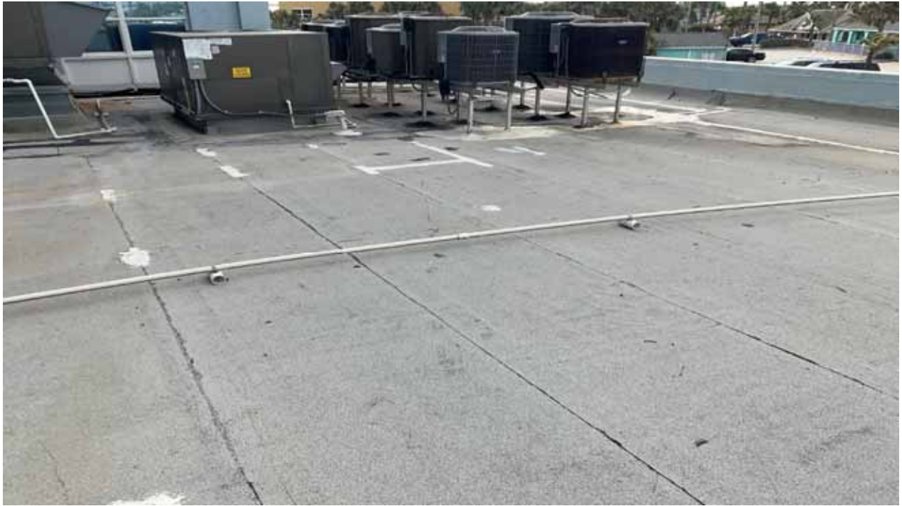
Roof - Lower South
