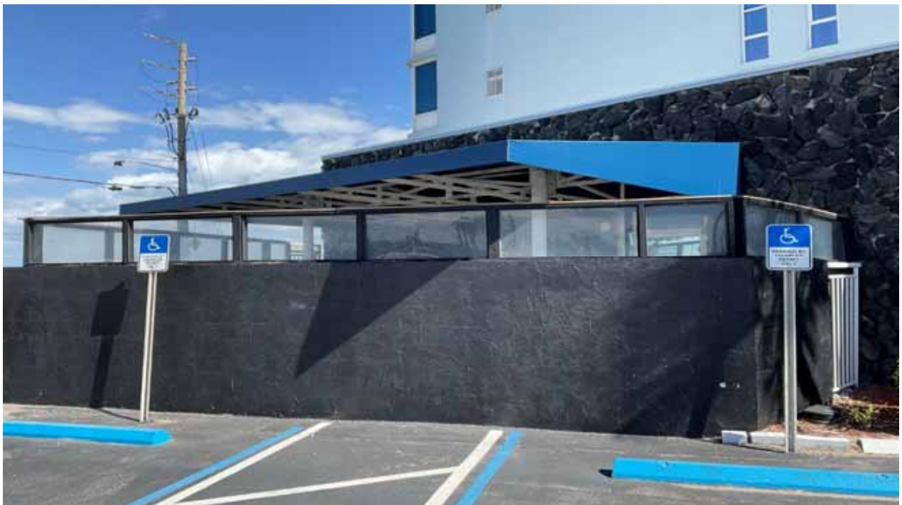
Awning - Break Area
