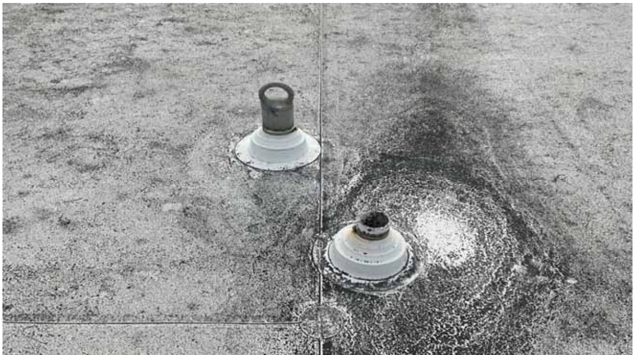
Roof - Anchor & Plumbing Vent
