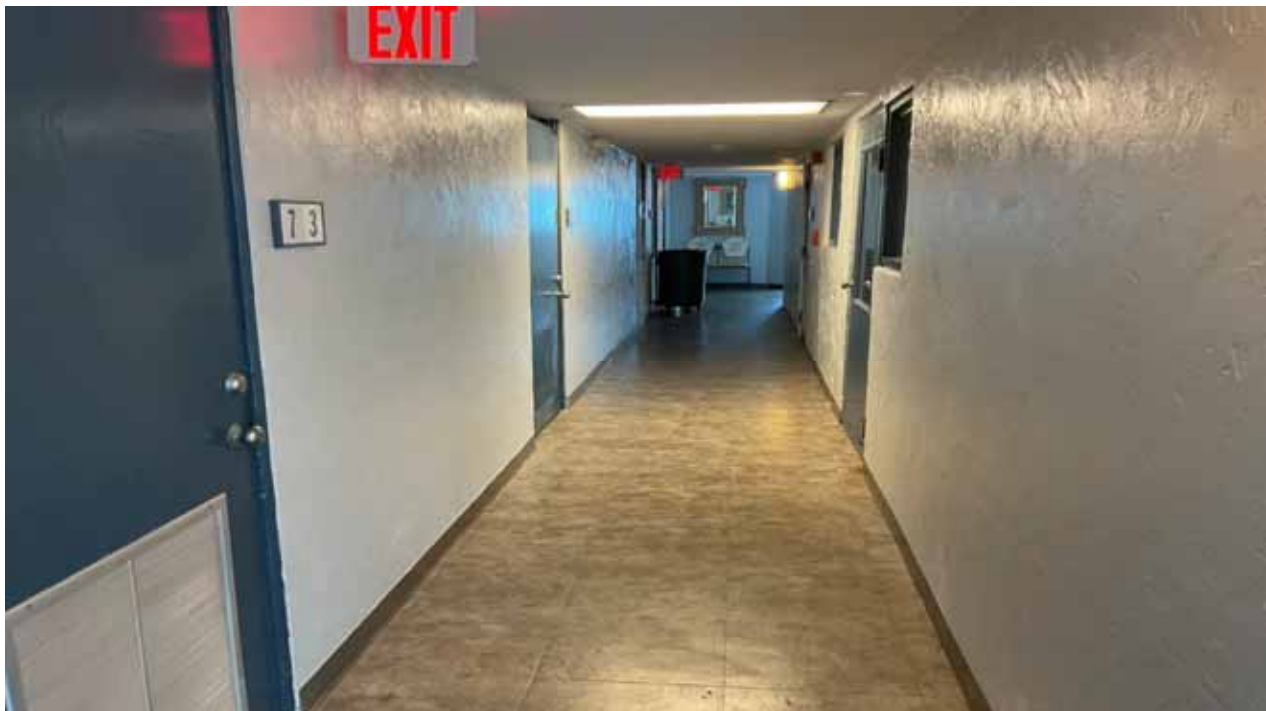
Elevator Lobby - Typical
