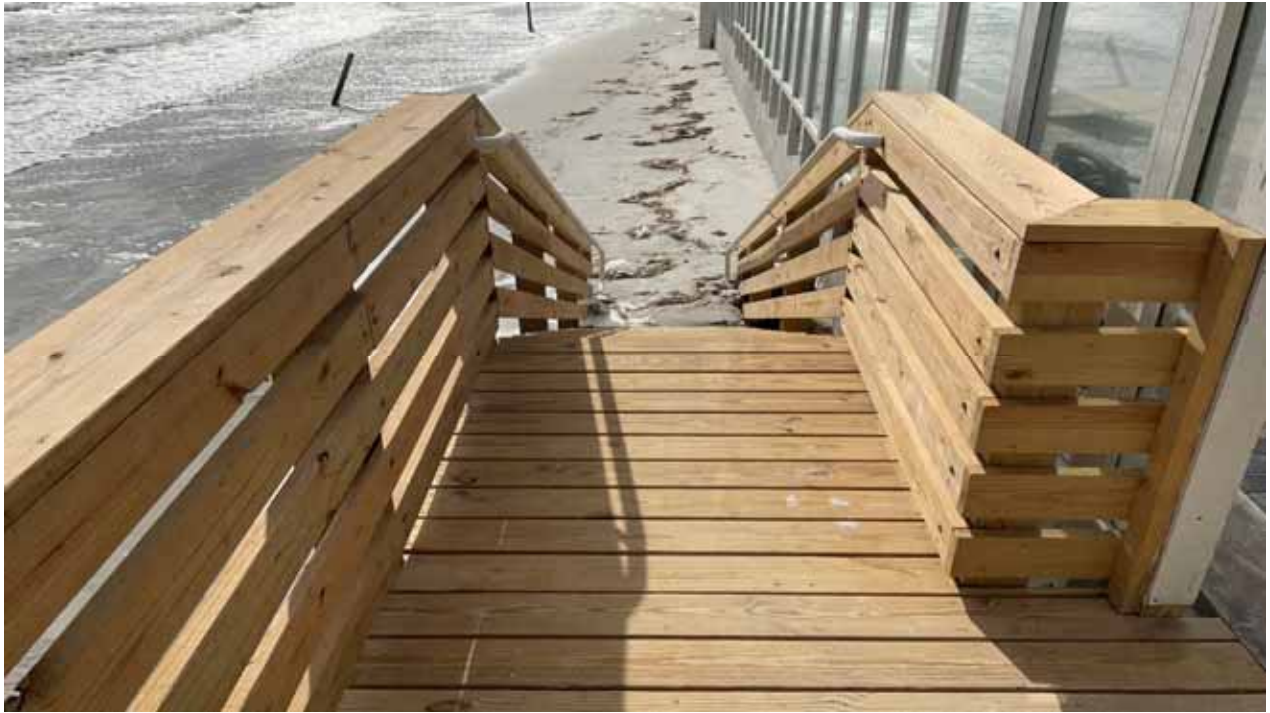
Stairs - Beach Access
