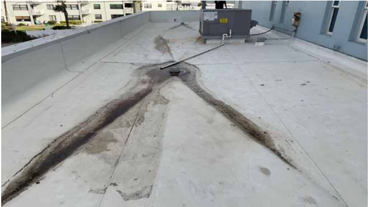
Roof - Lower North
