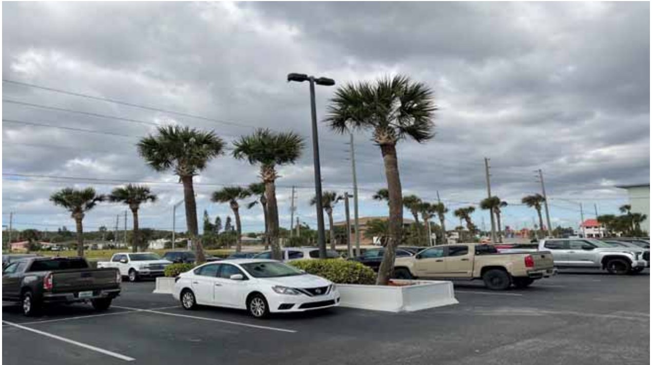
Lighting - Parking Lot
