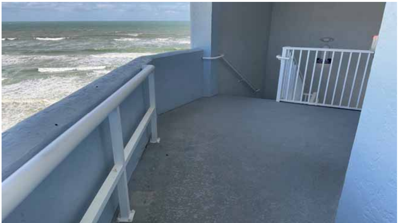
Exterior Walkway - North
